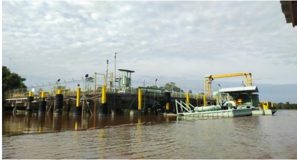
Water Intake PT. RAPP
